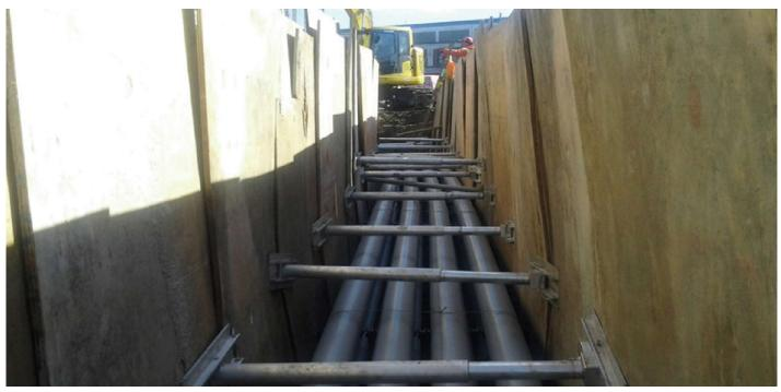
Crews will ready roadways and install an underground duct bank in which the new cable will be installed. This may include trenchless installation methods.
