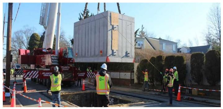
Underground vaults will be installed at intervals along the route to splice or tie together underground cables.
